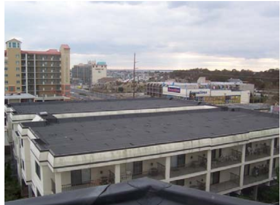
Photo 3 - Single ply roofing system - adhered
