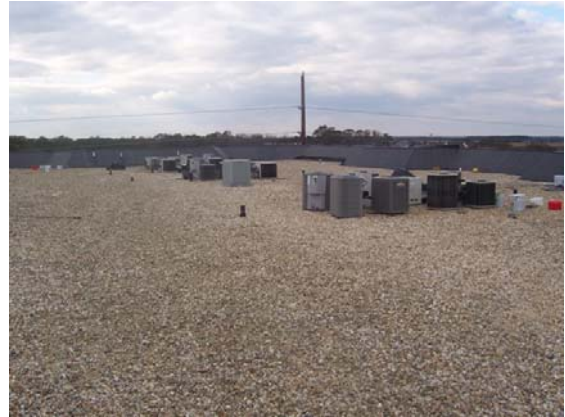
Photo 2 – Single ply membrane roofing
