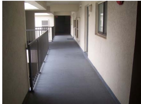
Photo 2 – Exterior walkway coated
