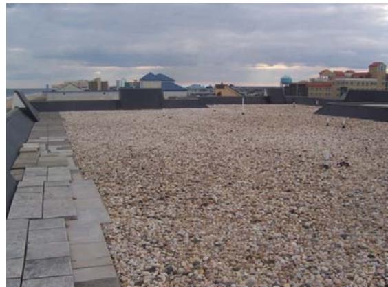
Photo 3 - Single ply roofing system - ballasted
