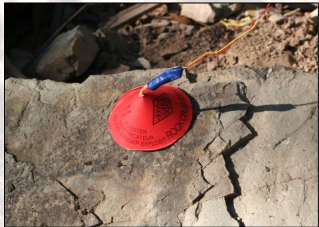
RDX 'Rock Crusher' shape charge with blasting cap
