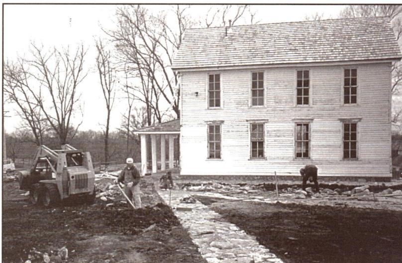
Restoration in process at Mt. Gilead School
