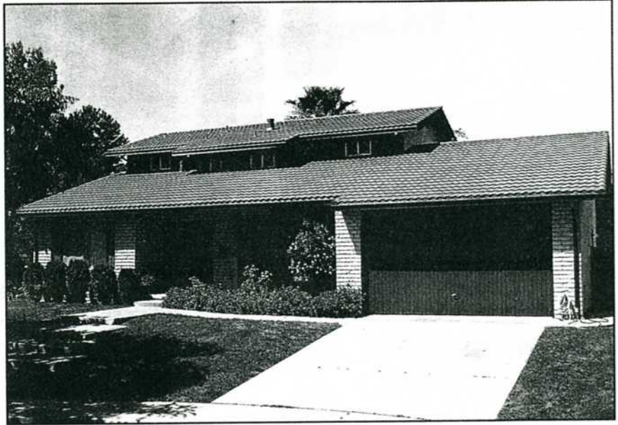
Stone Coated Steel Tile on the home of Mike Devlin; Assistant Fire Chief, City of Alameda, CA
