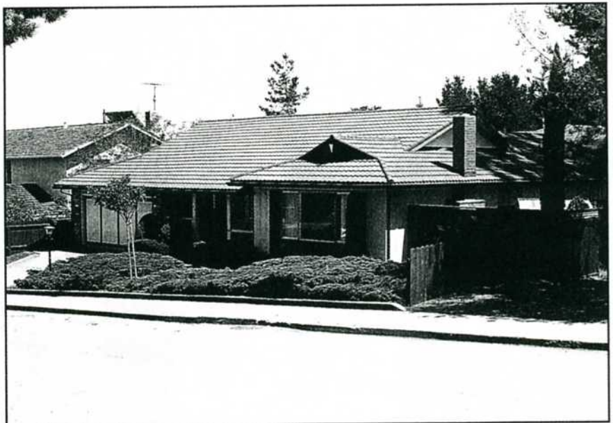
Stone Coated Steel Tile on the home of Victor Mangini; Past Mayor, City of Burlingame, CA.
