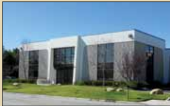
AGMillworks Factory and Offices in Ventura, California, USA
