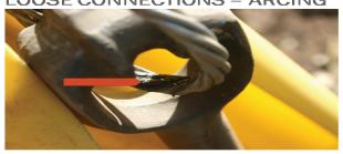
The design allows for ground current caused by a system disturbance, to flow in one anchor and out another because two down guys are tied together with a common metal bolt creating a path for Electrical Current to flow. With this design, current can also be caused just from induction from the 69kv line under heavy loaded conditions.
