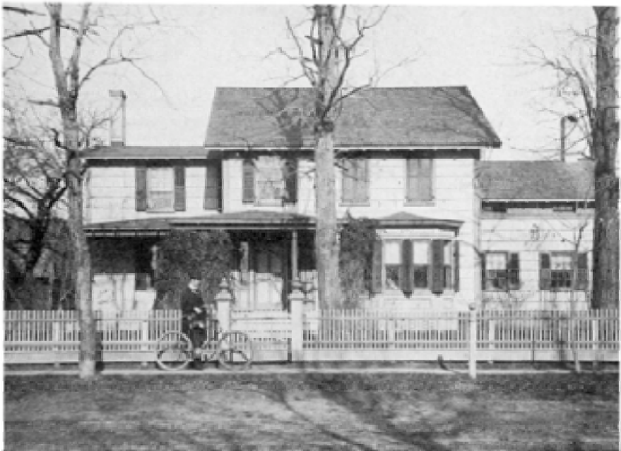
About 1911. Note bay window which was later removed.
