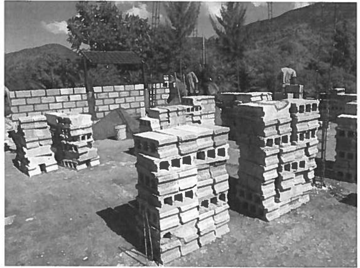
Starting construction on second floor to the school.
