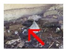
Waste line leaks which are visible from under the house (in the underfloor crawlspace) were noted at the master bathroom shower drain.
