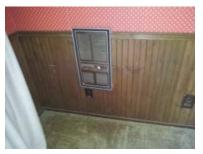
The unit at the downstairs bedroom has no control or thermostat, therefore it is not functioning either. That means that this bedroom has no means of heating.
