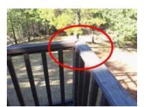
Many surface board fasteners are loose.
