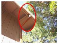
Debris (from overhanging vegetation, mineral deposits from roof shingles, etc.) was noted in the gutters, this is a common condition, however it will accelerate deterioration of gutters. Gutter cleaning is a preventative maintenance procedure which should be performed at least once a year.
