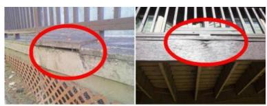
Wood fungus was noted to the surface boards or framing at the underside of the porch. Wood fungus is the first stage of dry rot, and
