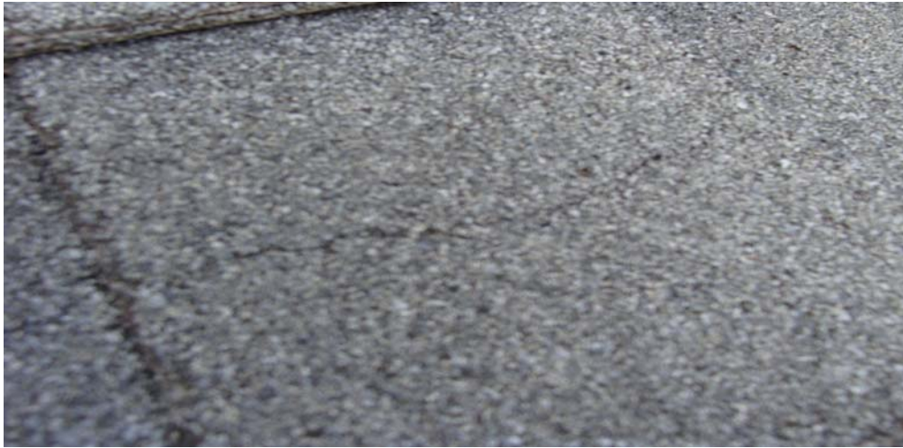
cracking of the composition shingle.
