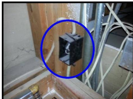
No junction box cover
