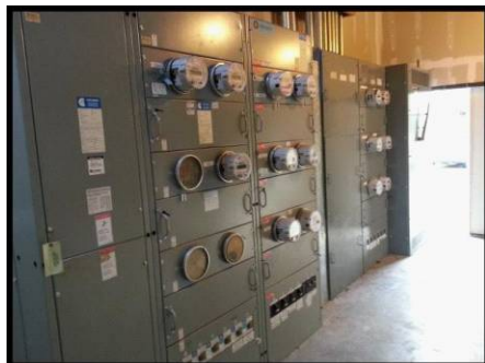
Panel #1 - Main Panel/Switchboard
