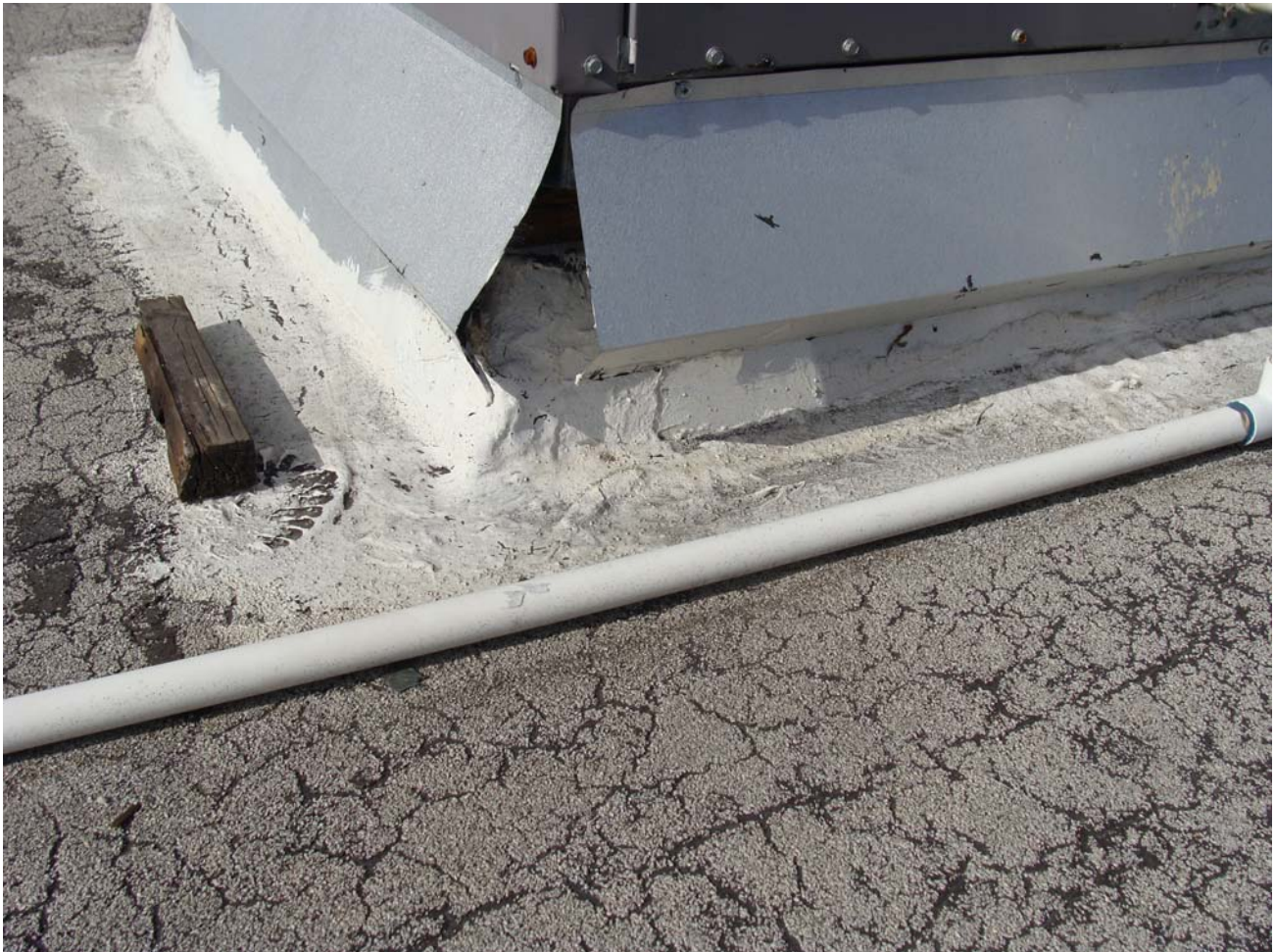
This photo shows an improperly flashed mechanical unit as well as the cracking or aligating of the mineral surfaced cap sheet.
