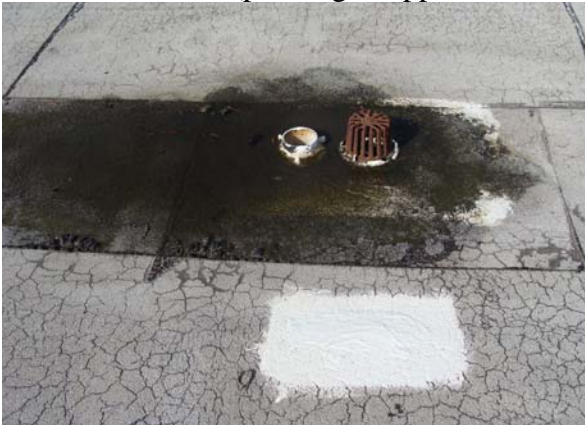
Compression drain and overflow
