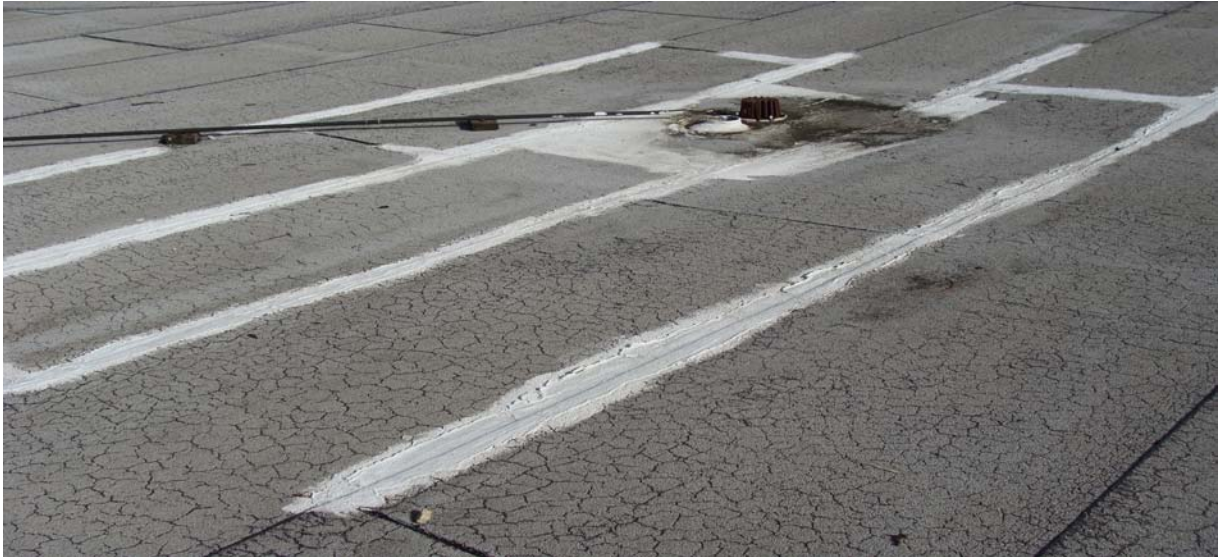
More repairs using elastomeric paint or coating at the seams in the cap sheet.
