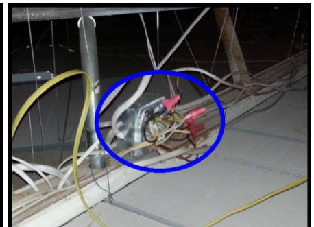
No junction box cover
