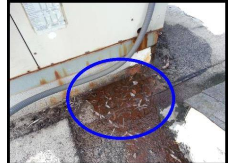
Condensate drain stains on roofing surface
