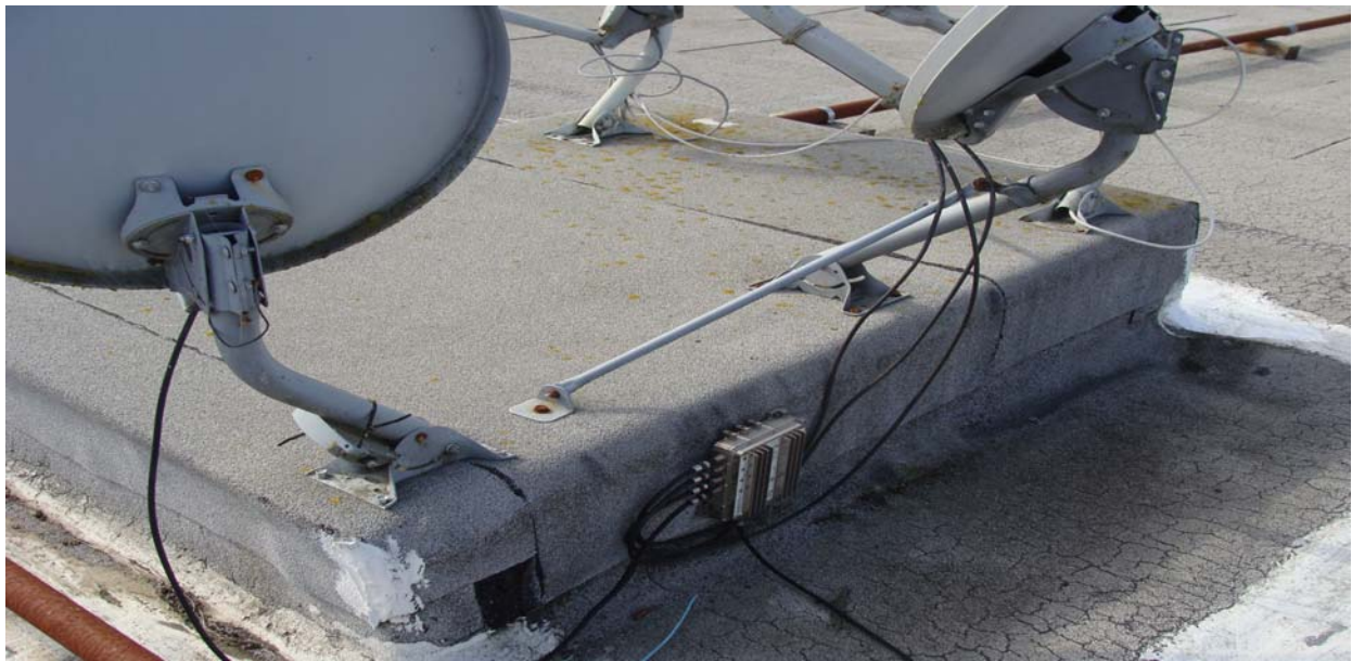
Improperly fastened satellite units
