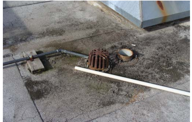
Condensation lines from A/C units at drain
