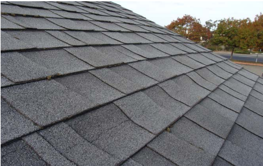
More crack in the Composition shingle roof.
