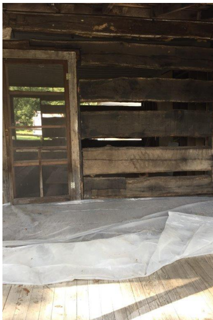
August 30 – with the south porch logs exposed and restored, new chinking was added.
