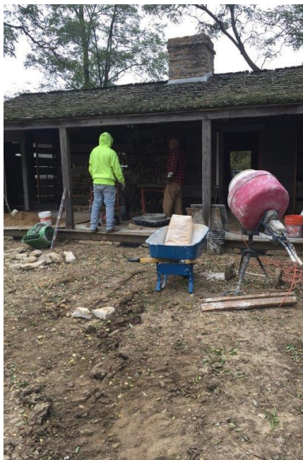
August 30 – with the south porch logs exposed and restored, new chinking was added.
