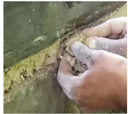
Replacing the chinking and daubing between the logs. Pishny Restoration Services facebook page
