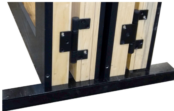
FIG 7: Support Bottom of Panels During Install
