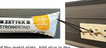
Apply glue to the bottom of the metal plate. Add glue in the holes in the floor. Make sure the holes don't overflow when you place the floor plate.
