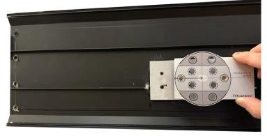
Use the metal template provided and measure the distance of the pins from the edge of the sill to find the placement of the holes in the floor.
