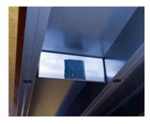
Use screws to apply pocket stops **FIG 13.** These must be removable in the event that future service is required on this unit.
