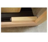
4 1/8" Bumper applied to bottom and top of interior sill and head jamb opposite of primary panel with handle set.
