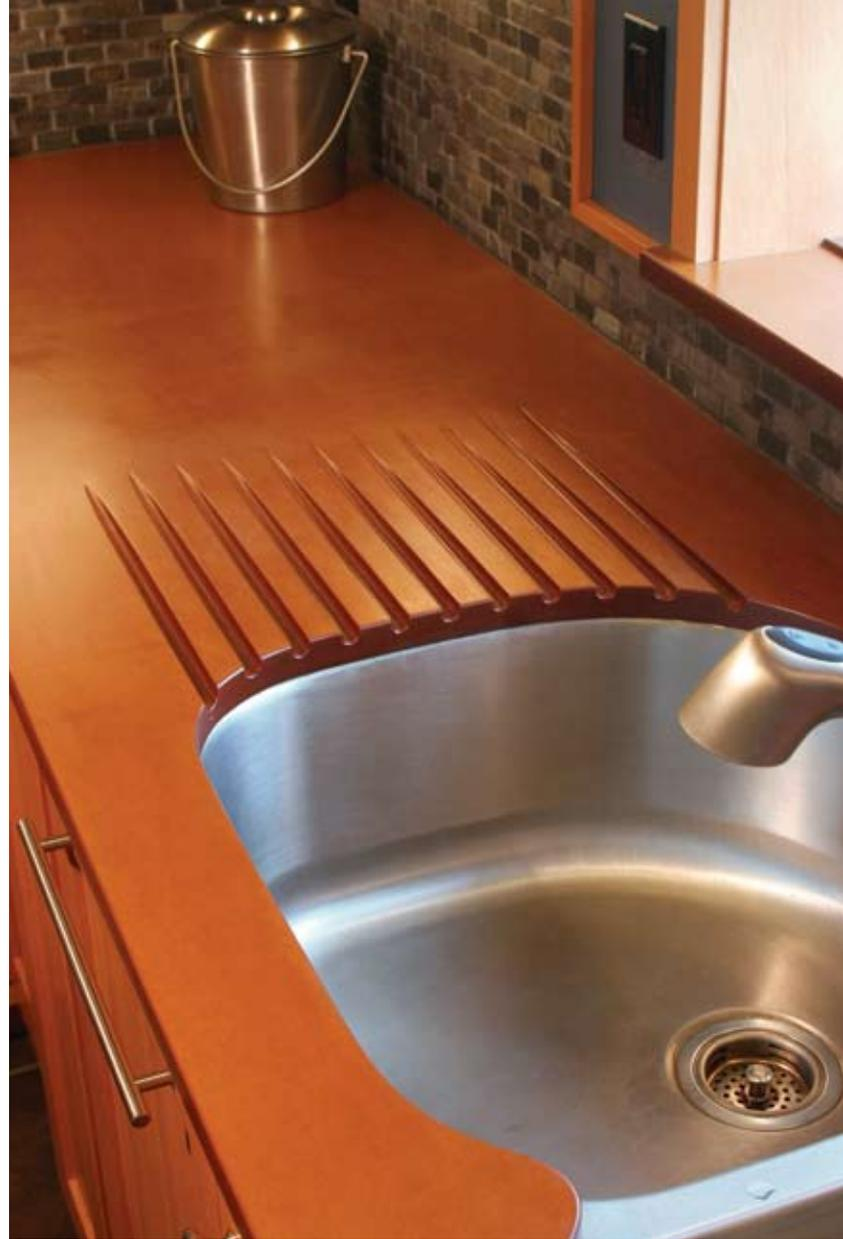
**Keeping dry.** Using a core-box bit on a sloped ramp, reviewer Dan Meyers milled the tapered slots in this PaperStone countertop to make an integral drainboard. This is the 1-in.-thick material in the color called leather.
