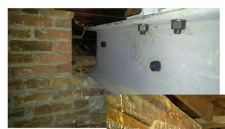
These images show the truss repair. The steel you see in the top picture is replacing the broken piece of truss that you see
