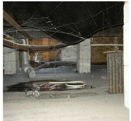
opened up for evaluation. The sub-floor insulation will clearly need to be replaced, but there may also be hidden conditions beyond that: Among these could be wood rot to the sub-floor or floor joists, infestation of wood destroying insects and even mold. All from one leaking pipe.
