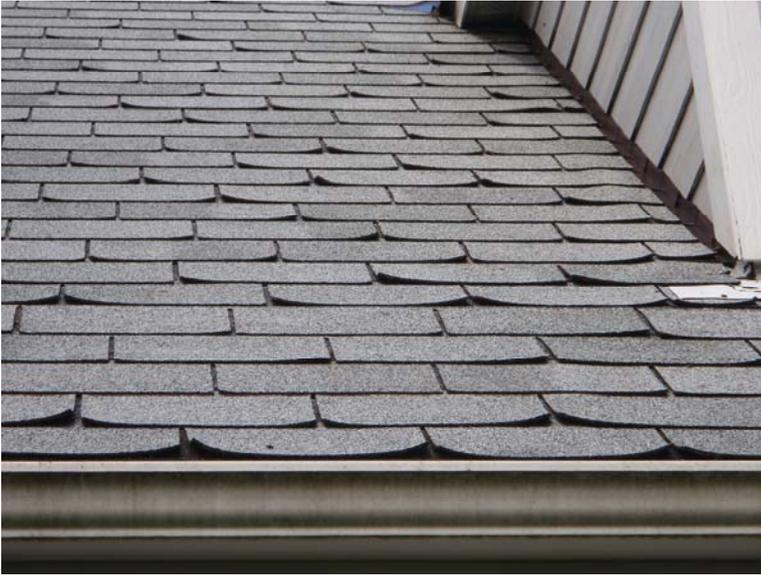
The picture at left shows a roof which failed after 5 years and had to be replaced – all because of inadequate ventilation.
